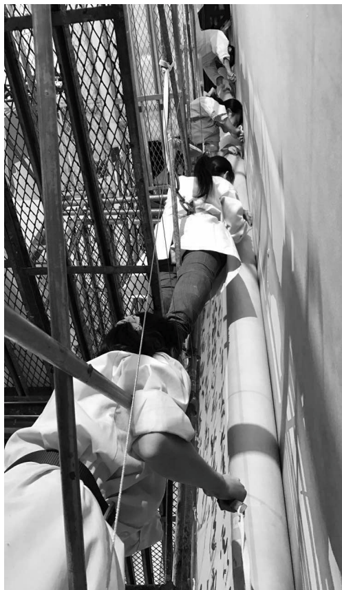
Figure 18. Coordinating removal from ceiling to floor
