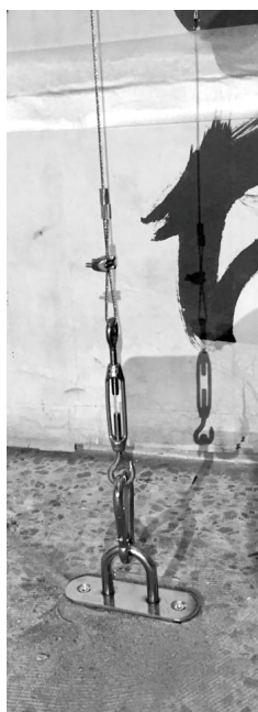
Figure 8. The floor attachments of the protection net
