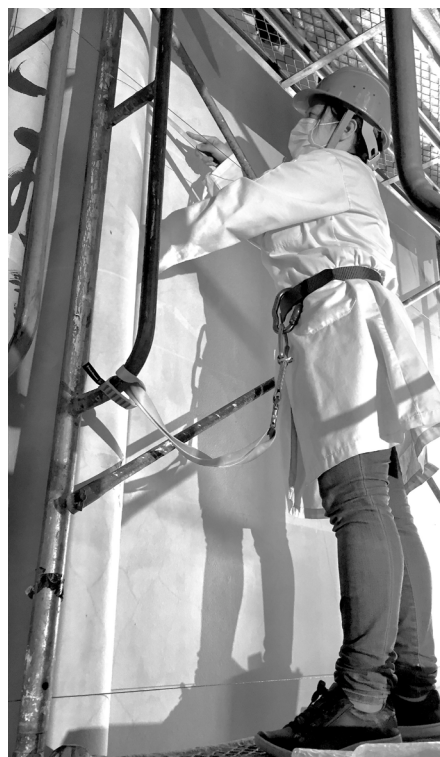
Figure 16. Moving safely on the scaffolding with quickdraws and safety harness
