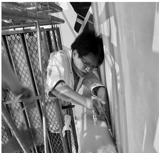
Figure 19. Working across lev- els to keep the line of removal straight, often in unusual positions
